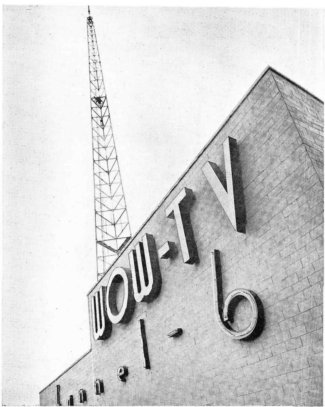
FIG. 1. Closeup view of WOW-TV showing the tower which supports the three-section Super Turnstile Antenna. The antenna has an effective height of 590 feet above average terrain. The location of the microwave relay receiver can be seen at the 270-foot level in the tower. Remote control equipment in the transmitter room permits 360° rotation as well as vertical tilt of the dish.
