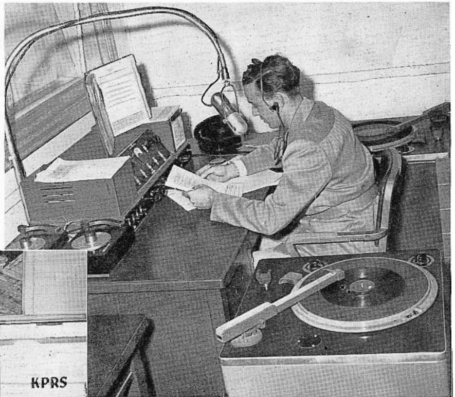
FIG. 4 (above). In the KPRS Studio Control Room are located two RCA 70-D Turntables, console and two 9JY RCA "45" record players.
